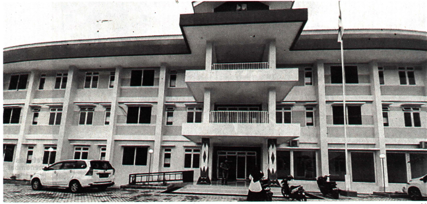
Rusunawa Bener Tower II.
